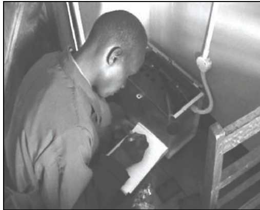
Figure 15: CHESCO technician checking the battery specific gravity
